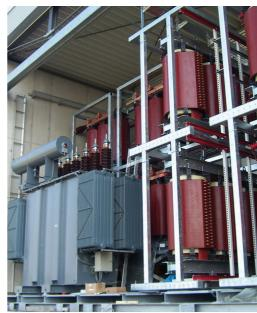
PSM Transformer Arrangement | The PSM transformer provides the AC power to each PSM module in the switching module assembly of the HVPS units.
